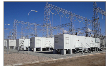
Dynamic energy solutions for a smarter grid
