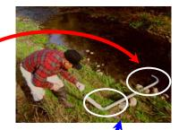
• Use Long-Sweep Elbows (PVC conduit fittings) to ease cable deployment through conduit for riverbank monitoring of flow / level in open channels.
